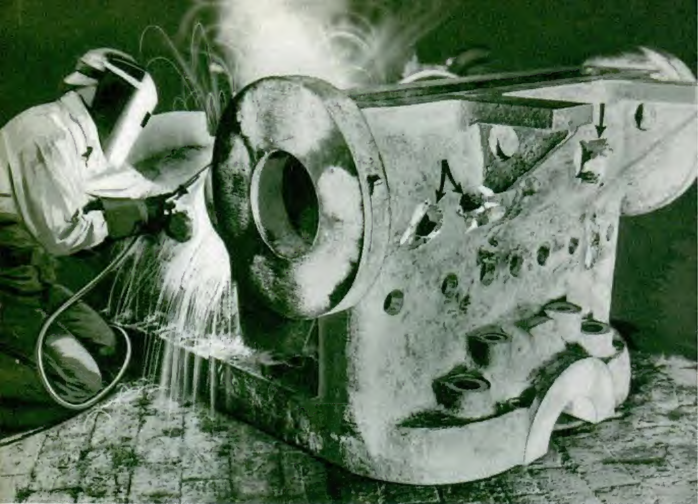
A welder fills in areas chipped from steel turbine casting (note arrows) after gamma rays had detected air-bubble flaws in steel
